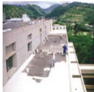
**LIMIX PlastiCoat 120** must be applied over 5 °C, and at + 20 °C **LIMIX PlastiCoat 120** stiffens enough to allow traffic after 24 hours.
